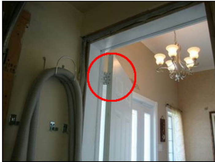
Install Self-Closing Hinge.
