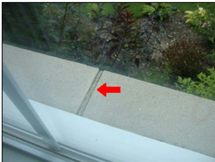
Repair Joint In Window Sills.
