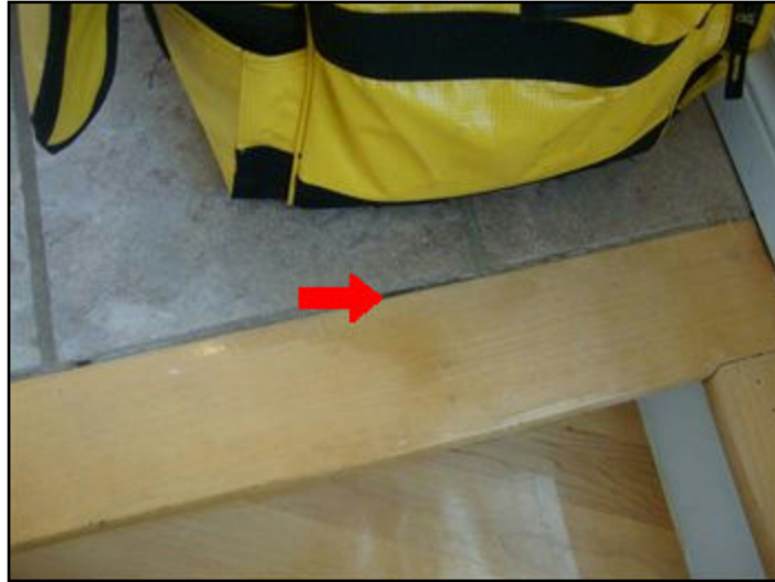
Seal Joint With Caulking
