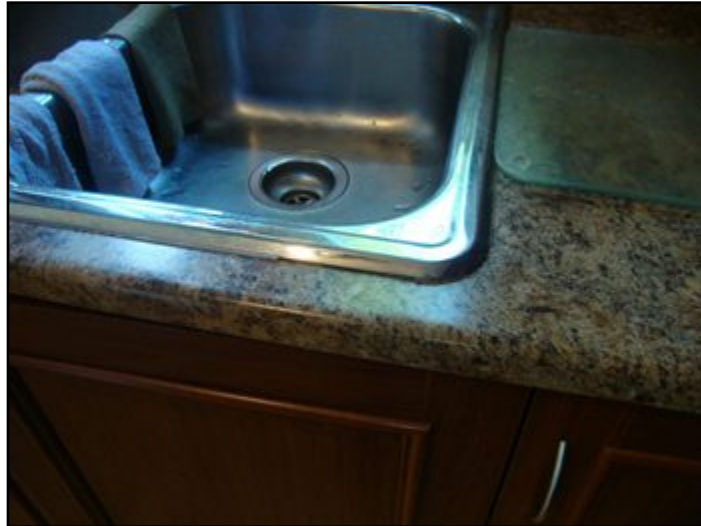
Caulking Repairs Around Sink.
