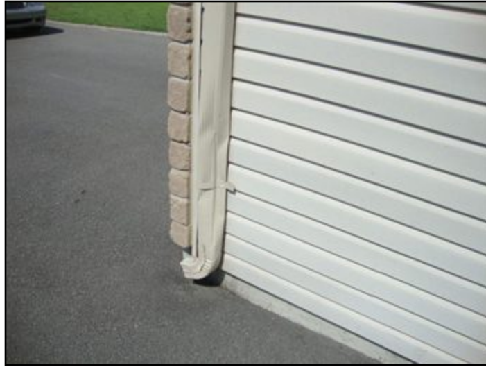
Damaged Downspout.
