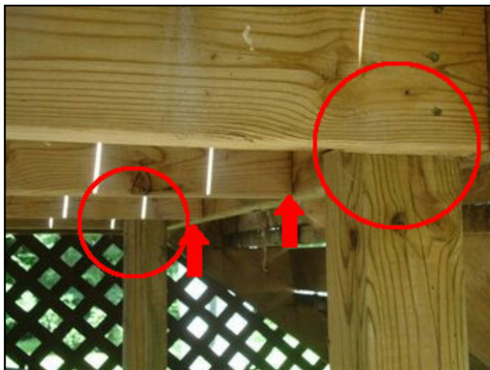
Brackets Could Be Added To Deck.
