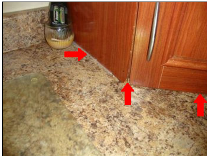
Seal Joints With Caulking.
