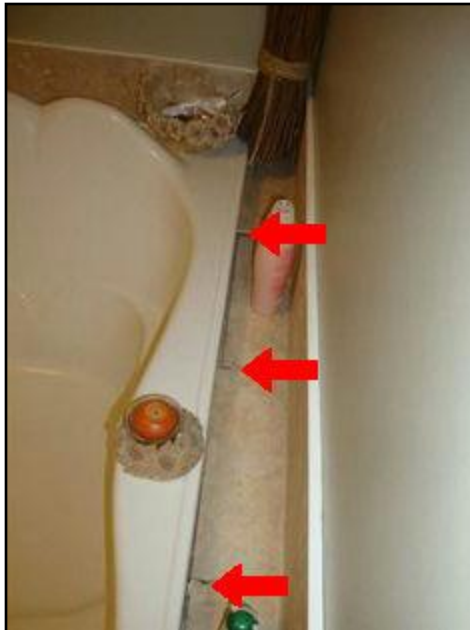
Missing Grout.
