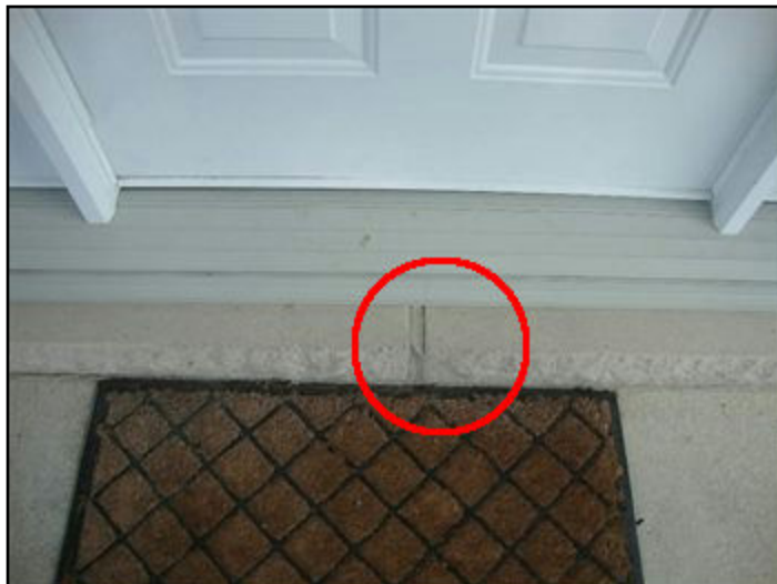
Fix Joint In Door Sill
